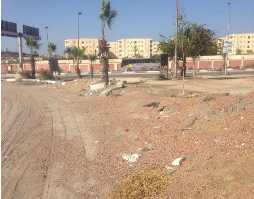
Figure (4-47) shows the road cross intersections
