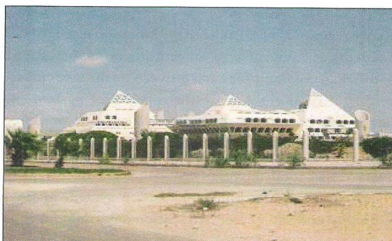
Figure (4-25) C-SAT in New Borg El Arab City (Temporary E-Just Campus)
