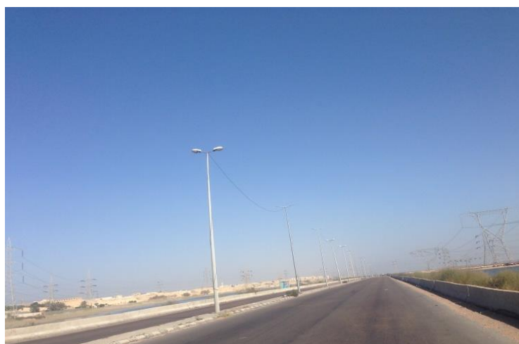
Figure (4-46) shows the current shoulders and medians
