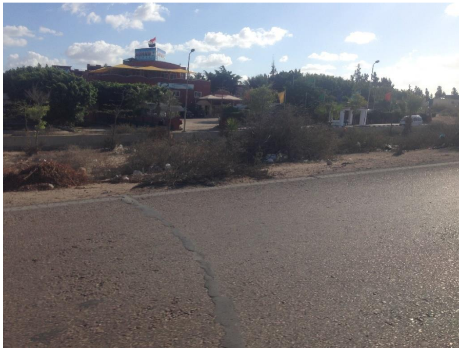
Figure (4-52) El Kafoury road
