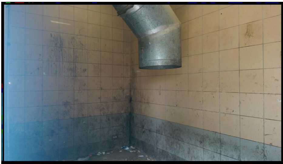
Figure (4-66) shows tube reaches the terminal building to the ground floor where the assembly room of solid wastes is located.
