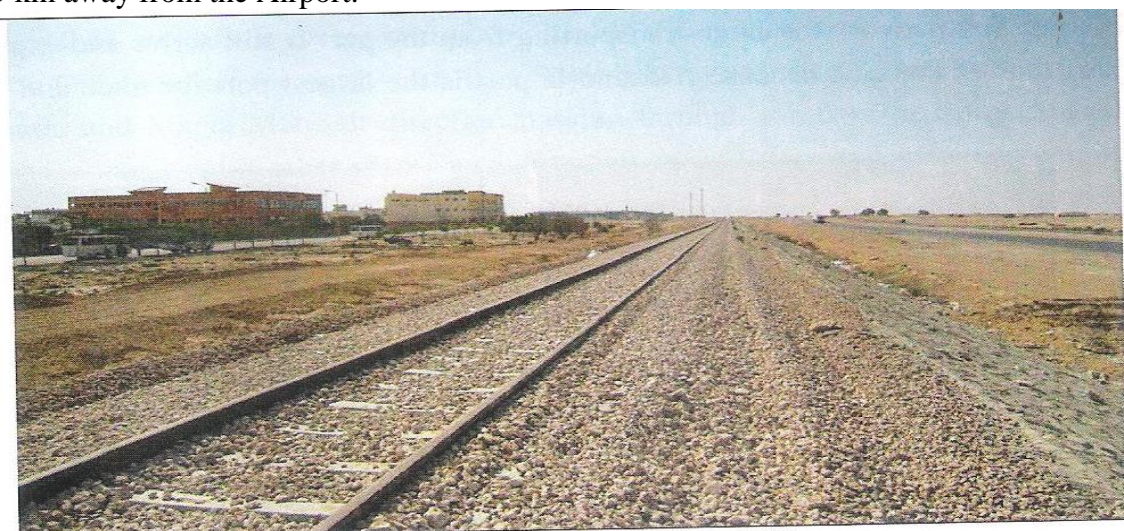
New rail truck in New Borg El Arab City (Industrial Area)
