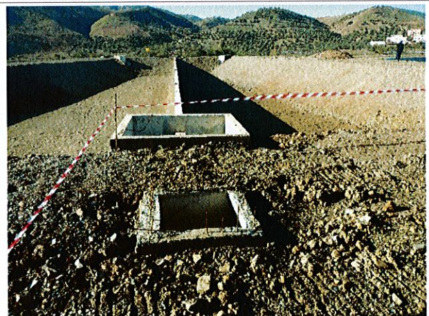
Completed sedimentation basins
