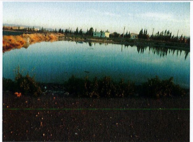
Basin maintained in operation
