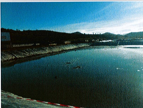
Basin maintained in operation
