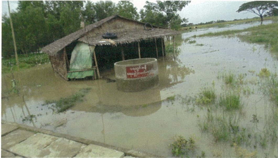
Photo 3 – Flooding around a water well
