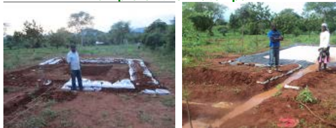
Embankment of water pan built with "Do-nou"
