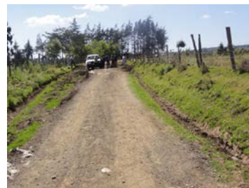
Photo 6: Road after repaired by CDF
