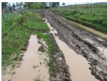
Photo 1: Road condition before repair
