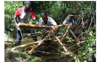
Installing a simple intake weir © E-COBSI
