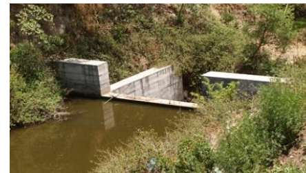
Irrigation facilities constructed in Himachal © JICA
