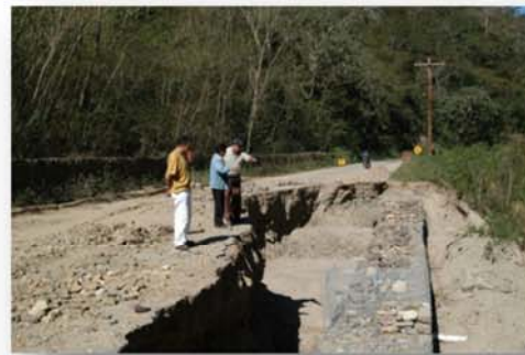
Damage on Route 7 after a landslide (Bolivia)
