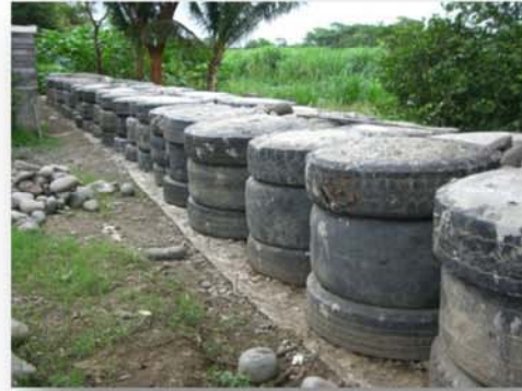
Walls using used tires (Costa Rica)
