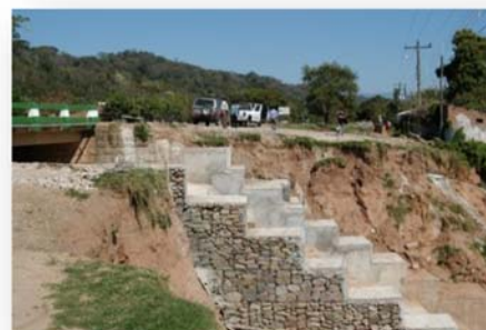
Shoulder protection works at National Road 7 in Bolivia
