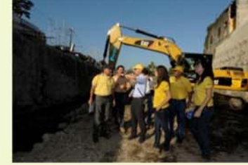
Inspecting reconstruction site after hurricane impact
