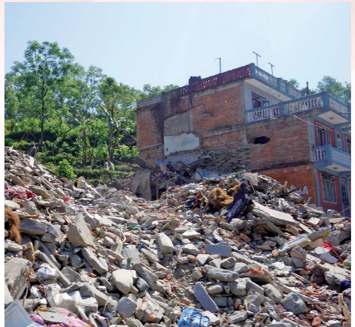
Examples of some buildings (in the back) that survived the earthquake by having, though inadequate, rebar and crossbeams. The collapsed private buildings did not have any reinforcements (foreground) (Nepal, May 2015)
