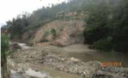
Slope failure in a road portion along Bagmati River near Kokhana during the 2015 Gorkha earthquake (after KUKL)
