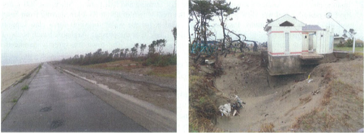
Fig. 39 (a) Damaged seawall and control forest and (b) Severe scouring at house's footing
