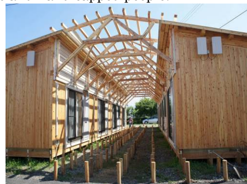
Picture 5 Temporary houses in Tono City (Iwate Pref.)
