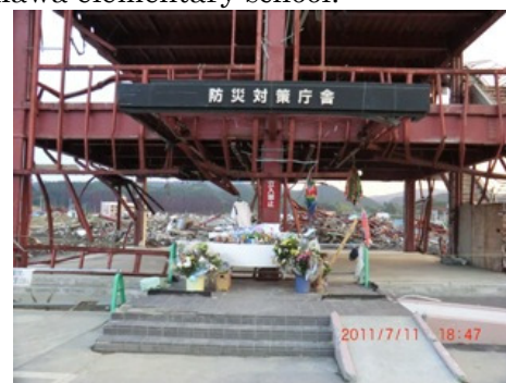
Picture 1 Minami Sanriku City disaster management office
