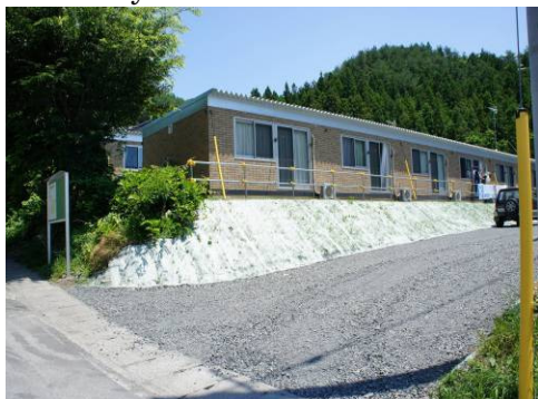
Picture 6 Temporary house in Otsuchi Town (Iwate Pref.)
