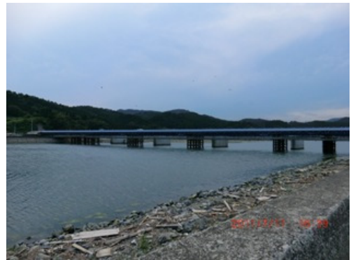
Picture 4 Temporary Kesen Ohashi (Bridge)
