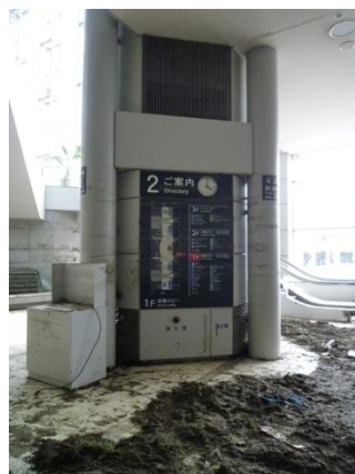
Terminal Building, Sendai Airport (Mar. 29, 2011 by Matsumaru)
