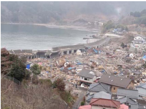
Photo 2 Sea wall collapsed and residential area was washed away
