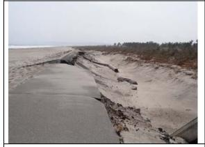
Collapsed Sea Wall. Tsunami Control Forest was mostly destroyed.
