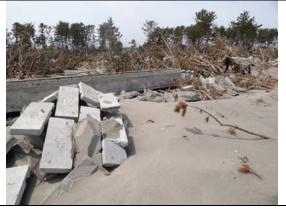
Debris of Sea Wall, located behind the original position.
