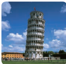
B The Leaning Tower of Pisa in Italy: It has a lean of 5° towards the south.
