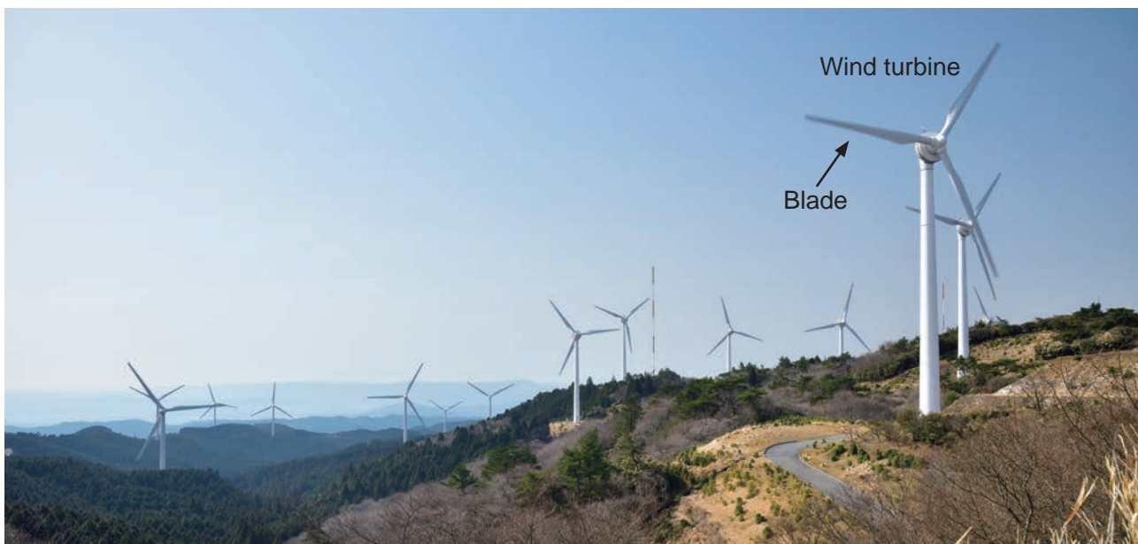
Wind turbines to generate electricity
