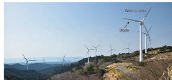
Wind turbines to generate electricity
