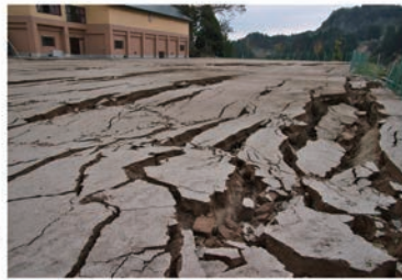
Earthquakes cause cracks on the ground.
