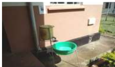
Hand washing facility installed in proper place
