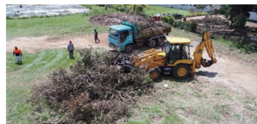
▲ Activities to remove disaster waste from the cyclone aftermath in Tonga.
