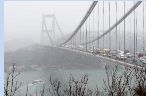
Fatih Sultan Mehmet Bridge (The Second Bosphorus Bridge) in Turkey
