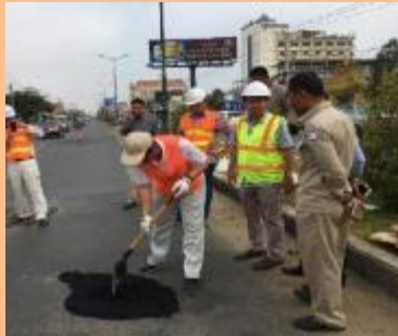
Repair of potholes using Excel Patch
