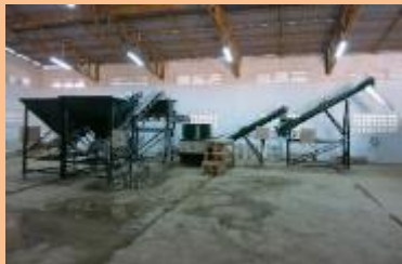
Production Plant of Excel Patch in Laboratory of RID
