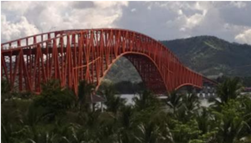
San Juanico Bridge
