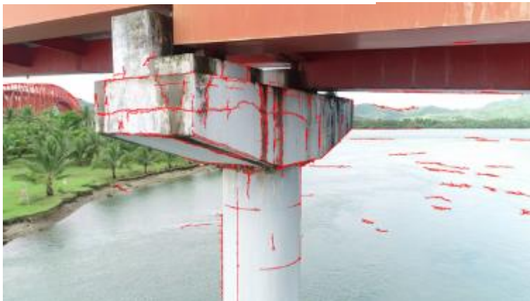
Cracks Identified by AI
