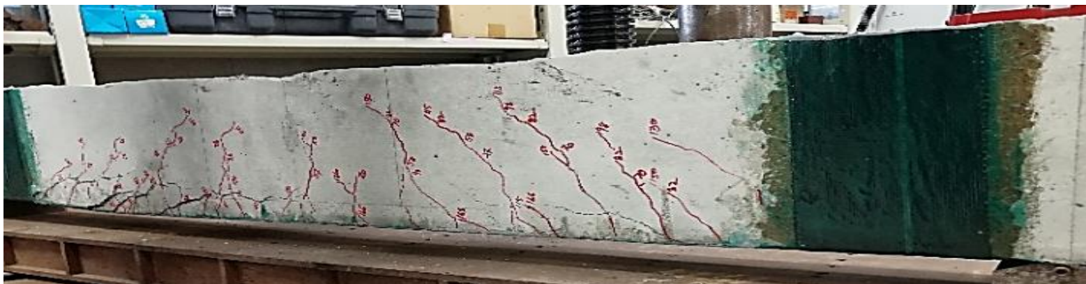
HS8F2A Failure modes=CS Crack nos. =25
