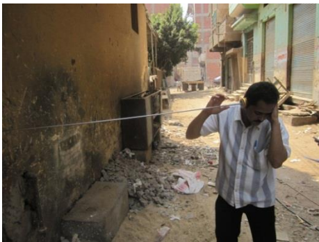
Photo-2: Leak Detection at House Connection
