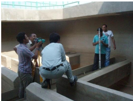
Photo-1: Adjustment of Trough Height
