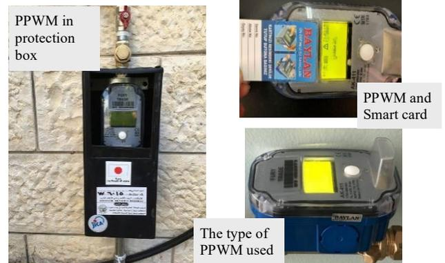
**The PPWM procured is ultrasonic type smart meter with a function of LoRa technology.** Twelve vending stations (VS) (Figure 13) were set up at convenient locations where customers could buy credits to recharge the meter. Through the Gateway and LoRa technology all PPWM could communicate remotely with PPWM server and PPWM customer database.
