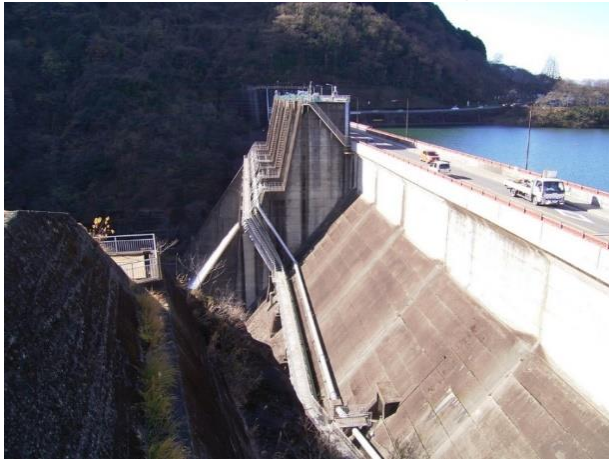
Multi purpose dam
