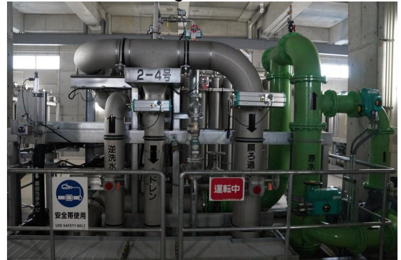
Inside of water purification plant “CERAROKKA”; built by PFI scheme in Yokohama
