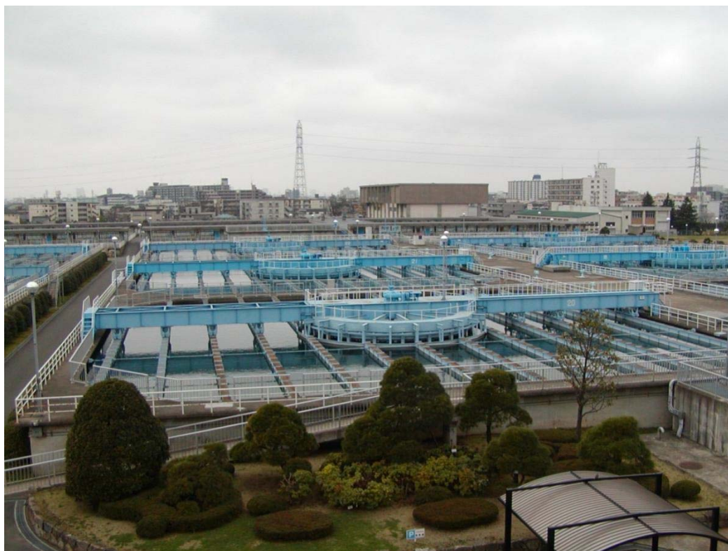
Photo 2. Kanamachi Water Treatment Plant, Bureau of Waterworks, Tokyo Metropolitan Government. It is equipped with advanced water treatment facilities which include rapid sand filtration, high-speed coagulation, flocculation and sedimentation reservoir. It also has power generation facilities, constructed using private financing (April 4, 2004).
