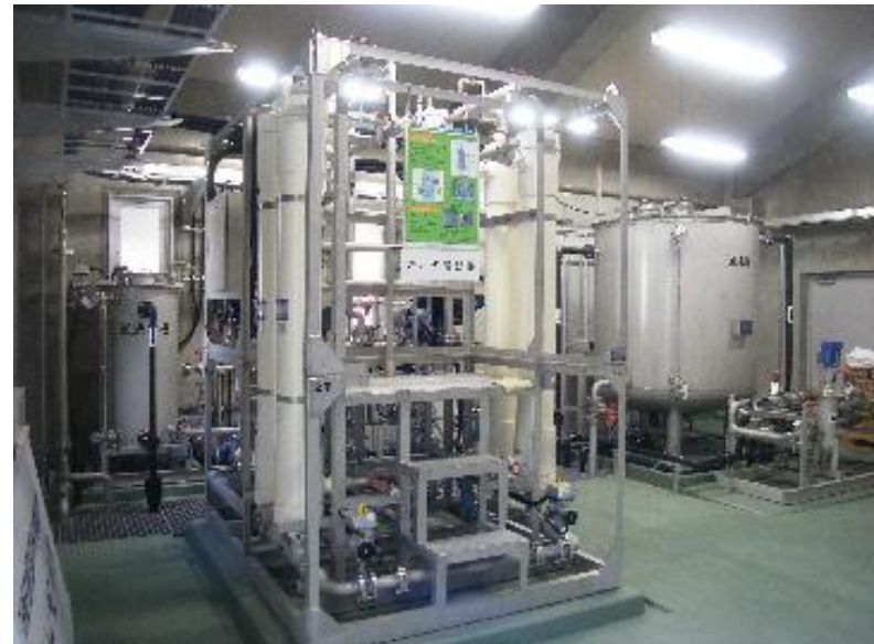
Membrane filtration facilities, Water supply system for Kuroda area in Kyoto city, Waterworks Bureau, City of Kyoto
