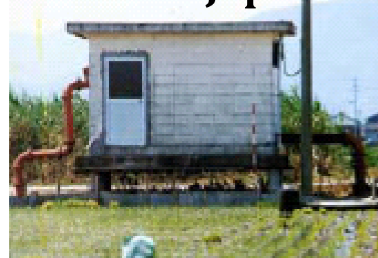
Lifting phenomena at pumping facility
