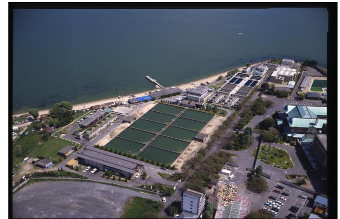
Yanagasaki water treatment plant, Otsu City Public Enterprise Bureau
