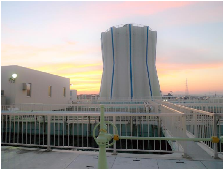
Elevated tank, Hachinohe Region Water Supply Authority
