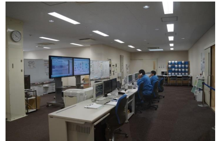
Kawai Water Treatment Plant by PFI Scheme, Yokohama City
