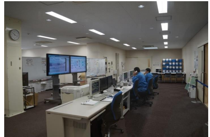
Kawai Purification Plant by PFI Scheme, (BTO) Yokohama City
