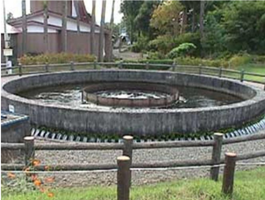
Cylindrical Siphon to allocate water equally, built in 1938 at Rokugou town, Akita Prefecture http://www.pref.akita.jp/fpd/tuchi/nanataki.htm
