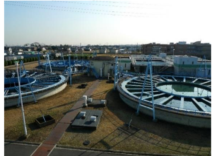
Kakinoki purification plant
