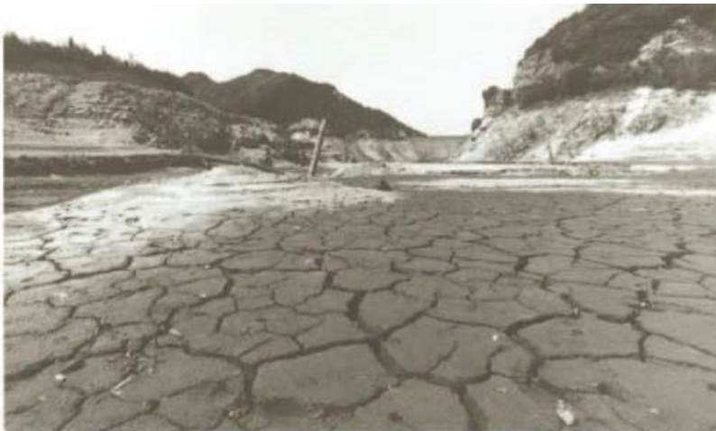
Parched Dam during Period of Abnormally Low Rainfall in 1978
