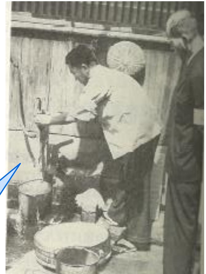
Staff repairing a tap
