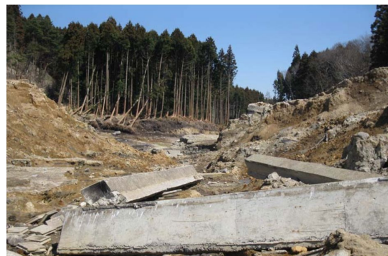
Source: Causes of the Break of Fujinuma Dam, Emergency debriefing one month after the great east Japan Earthquake by Tohoku University
