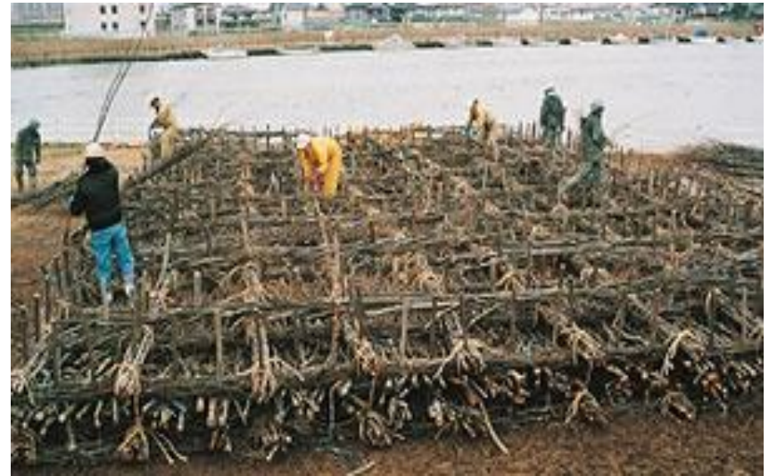
Riverbed and Riverbank Protection (Fascine Mattress)
