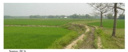
Figure 2.12 A Submerged Levee Protects Rice from Flooding (Haor District, Bangladesh)
