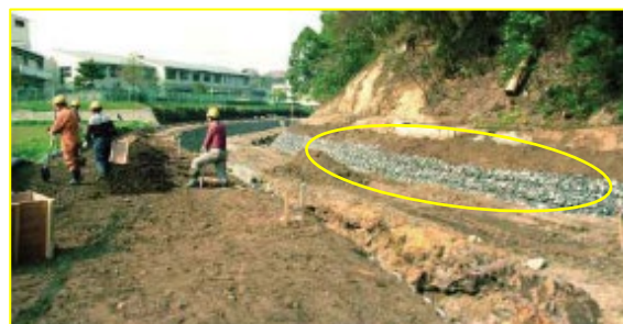
Renovation: gabion revetment on right bank
