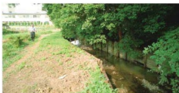
Before construction: plank hurdle revetment
