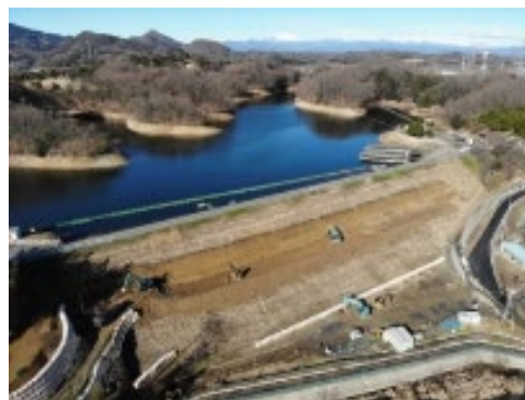
Figure 2.5 Seismic Resistance Reinforcing Works for Sannako Dam
