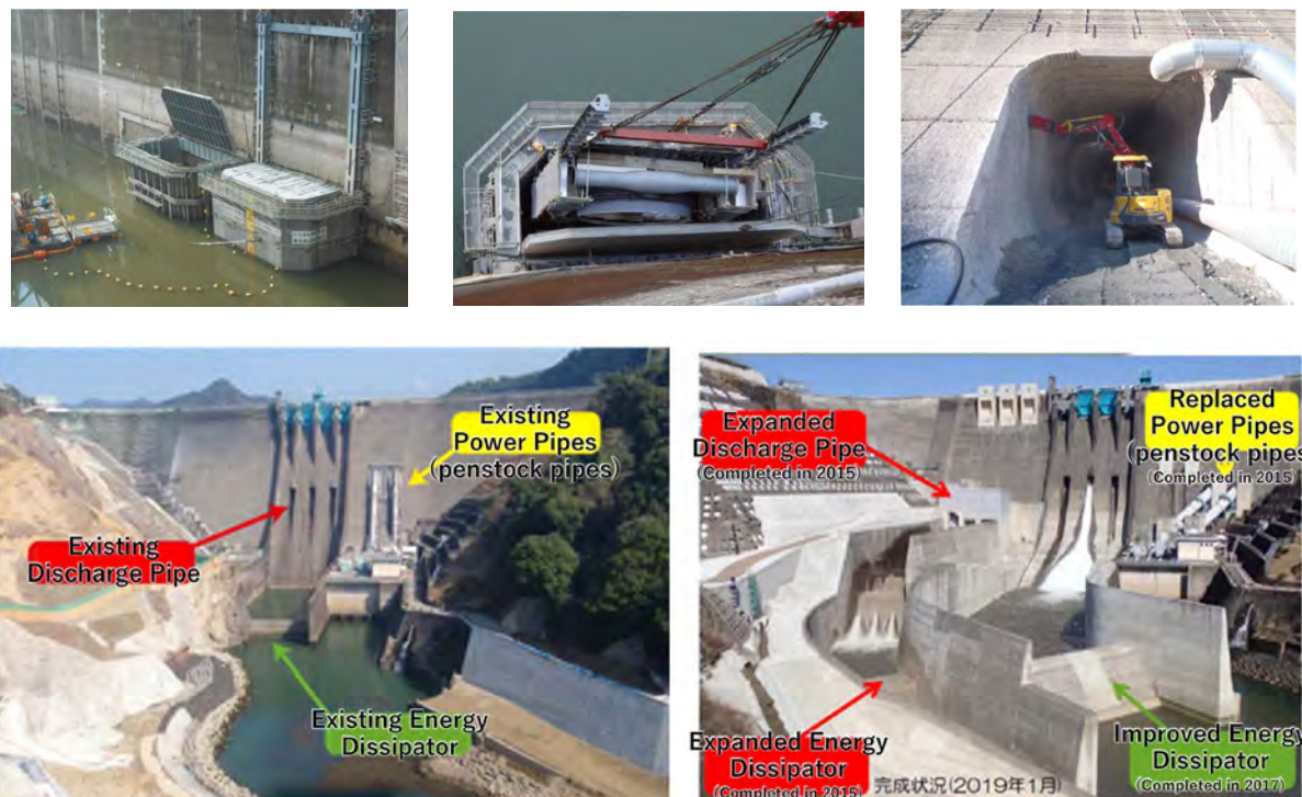
Note: (Upper left and center) upstream coffering, (Upper right) drilling of dam body, (Lower) before and after the works Source: Sendai-gawa River Office, MLIT
