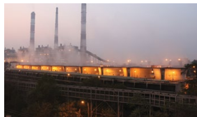
Bakreshwar Thermal Power Plant, West Bengal
