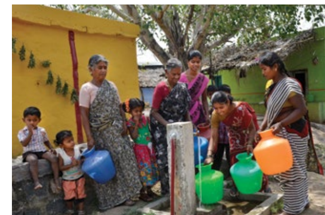
Safe drinking water point at Dharmapuri, Tamil Nadu under Hogennakal Water Supply and Fluorosis Mitigation Project
