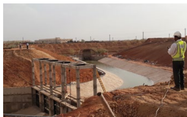
Work in progress at the Rajasthan Fluorosis Mitigation Project
