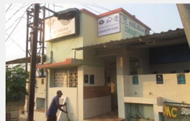
Community toilet constructed under Odisha Integrated Sanitation Improvement Project
