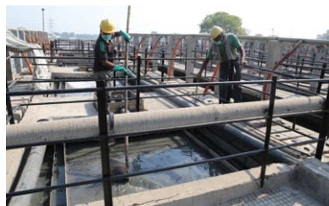
Cleaning of impurities from grid at Agra Water Treatment Plant
