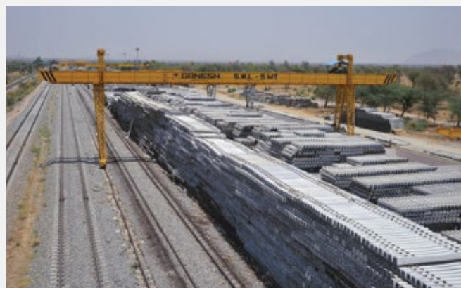
Work in progress at Dedicated Freight Corridor, Jaipur
