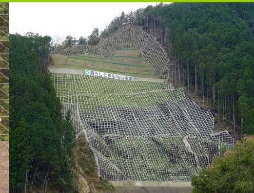
Image: Completed hillside crib work
