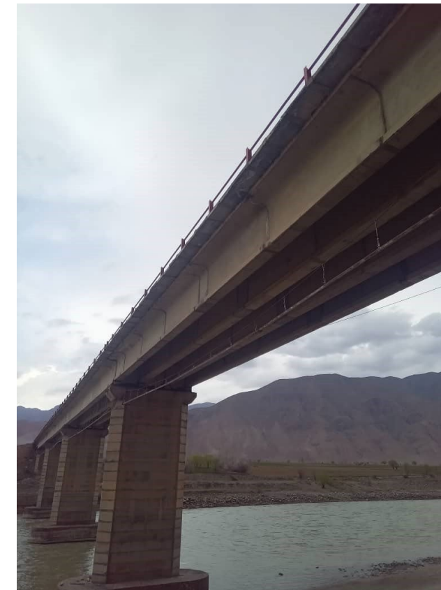
Condition of the bridge prior to reconstruction
