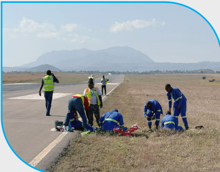
Airfield Ground Lighting (AGL) practical training session underway at Chileka International Airport, June 2025.
