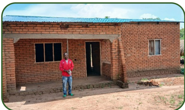
A house built from the proceeds of SHEP approach.
