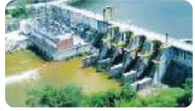
Construction of hydro power station with 72MW capacity in Upper Perak. (Completed 1983)
