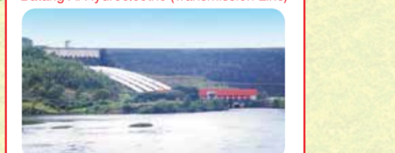
Construction of hydro power station and dual transmission lines. (Completed 1985)
