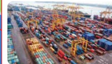
Constructed in 1973. Yen loan was used to fund the construction of sheet pile and main tie rod of the quay. (Completed 1973)
