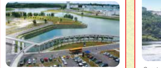
Building of the national university campus in Sarawak. (Completed 2007)
