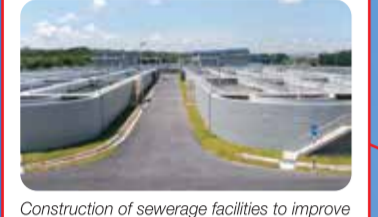
Construction of sewerage facilities to improve public hygiene and river water quality. (Completed 2009)
