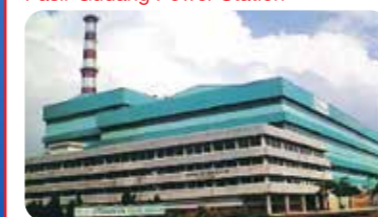
Construction of thermal power station with capacity of 240MW. (Completed 1982)
