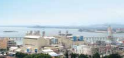
Port Dickson Power Plant
