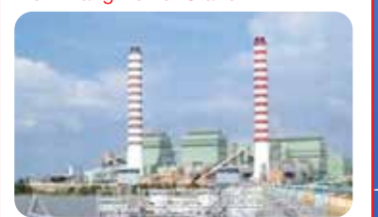
Construction of thermal power station with 2,400MW capacity. (Completed 2001)
