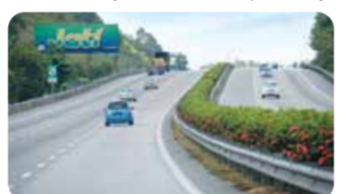
Improvement of Port Dickson interchange, construction of related roads and toll stations. (Completed 1987)
