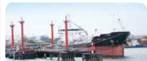
Construction of international port for shipping LNG and ammonia urea fertilizer. (Completed 1982)
