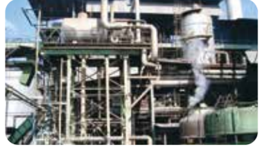
Construction of sugar processing plant in sugar plantation. (Completed 1973)
