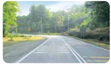
Improvement of Crocker Range Crossing Road between Kota Kinabalu and Sandakan. (Completed 1982)
