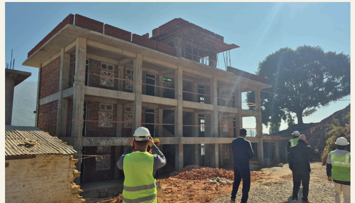
New structures being built for Masta Basic School, Bheri Municipality, Jajarkot
