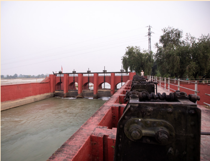
The well preserved old structures of the Irrigation System.
