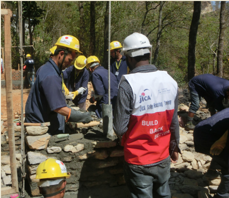
Mason training for House Construction in Sindhupalchowk
