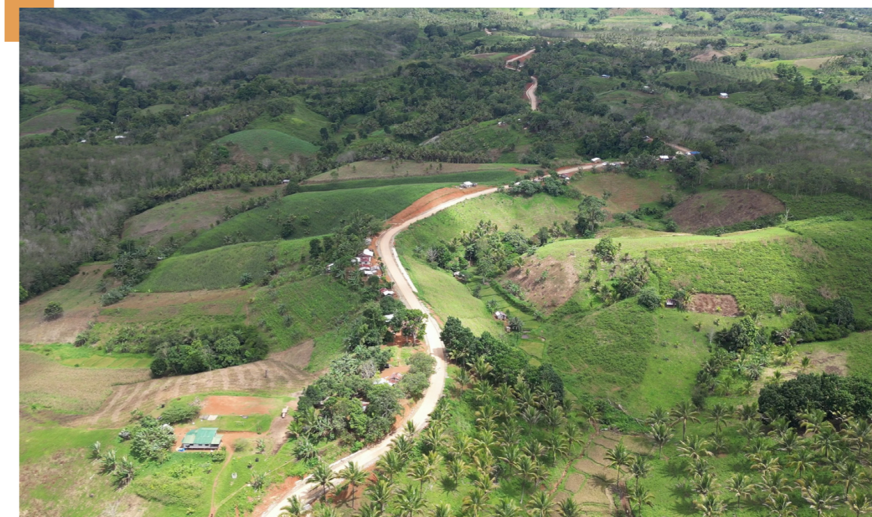
Completed 4.3km farm-to-market road in South Upi to improve connectivity of upland communities.
