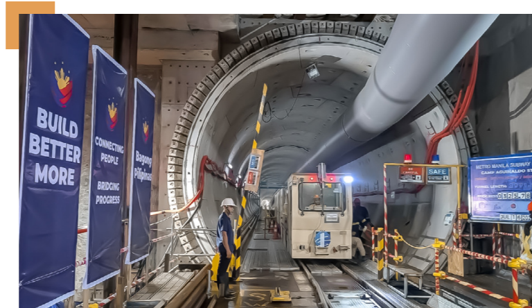
Metro Manila Subway Project, Camp Aguinaldo Station.
