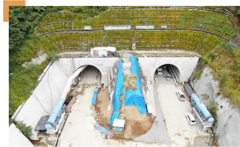
The twin tunnels of the Davao Bypass Road were successfully broken through.
