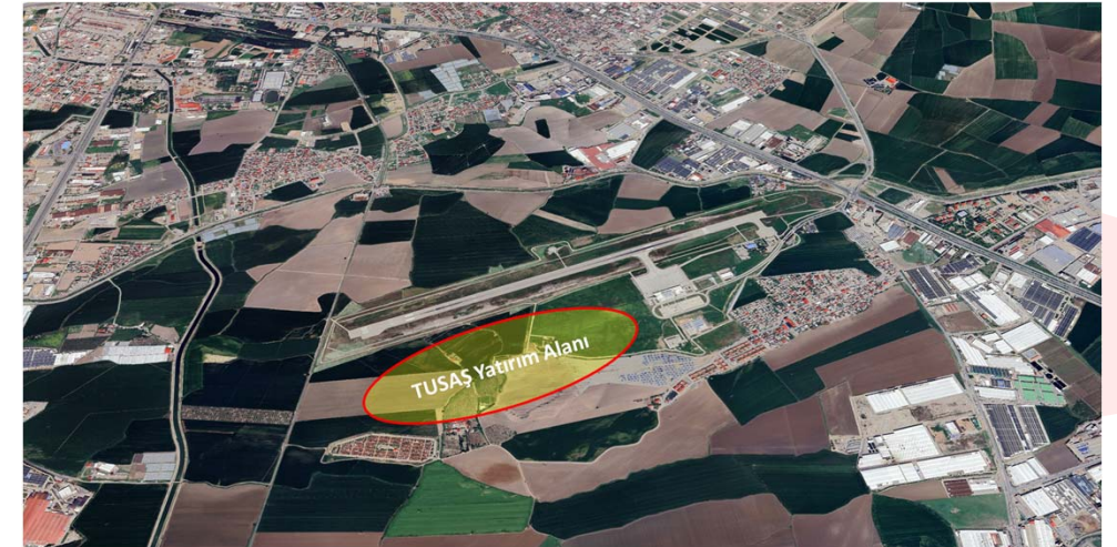
TUSAŞ Parts Production Factory in Kahramanmaraş
