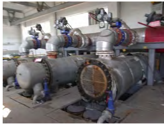
Heat Exchanger Units
