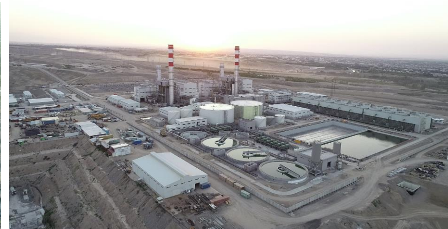
Turakurgan: Construction completed 2019
