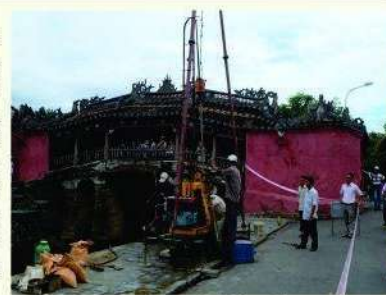
Geological drilling for infrastructure assessment
