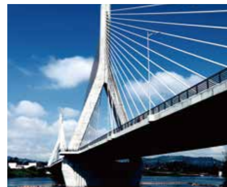
Construction of a New Bridge Across River Nile at Jinja (Uganda) Photo : The Zenitaka Corporation
