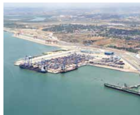
Mombasa Port Development (Kenya) Photo : Toyo Construction
