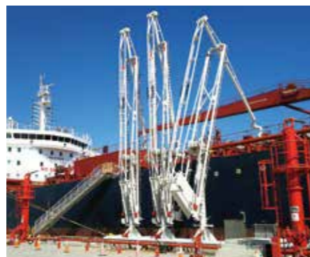
Nacala Port Development Project (Mozambique)
