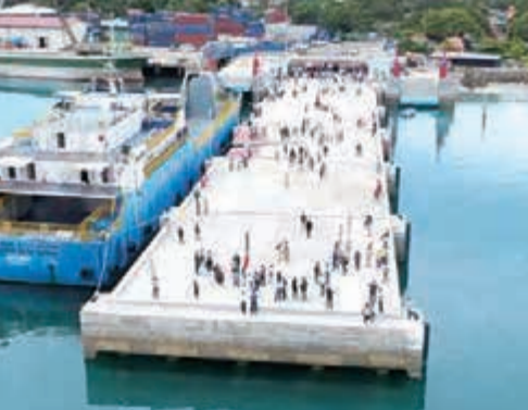
The Port of Dili, the country's only international port. The existing ferry terminal was relocated and expanded, contributing to the expansion of safe and efficient marine transportation (Timor-Leste)
