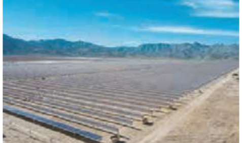
JICA signed a loan agreement with Infraestructura Energética Nova, S.A.B. de C.V. (IEnova), a Mexican energy company, for expanding its large-scale solar generation business and contributing to the efforts to combat climate change (Mexico) Photo courtesy of IEnova.
